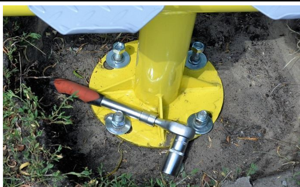
2. To mount the pole to the foundation you need: 4 normal galvanized washers (wide ones), 4 galvanized split washers, 4 16mm galvanized nuts and a no.24 wrench. All the washers and nuts are supplied with the device.
