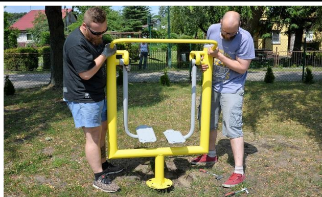
1. Position the device on the threaded bolts sticking out of the anchor in such a way as to not damage the threads.
